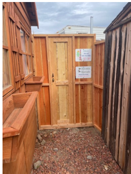
New Wall and a Door to Where?
