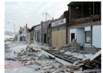
Earthquake Damage in Eastern Nevada, 2008
